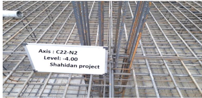
Figure no 2: Rebars used for implementing CEGE
