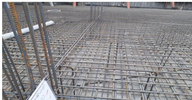
Figure no 3: Rebars used for implementing CEGE
